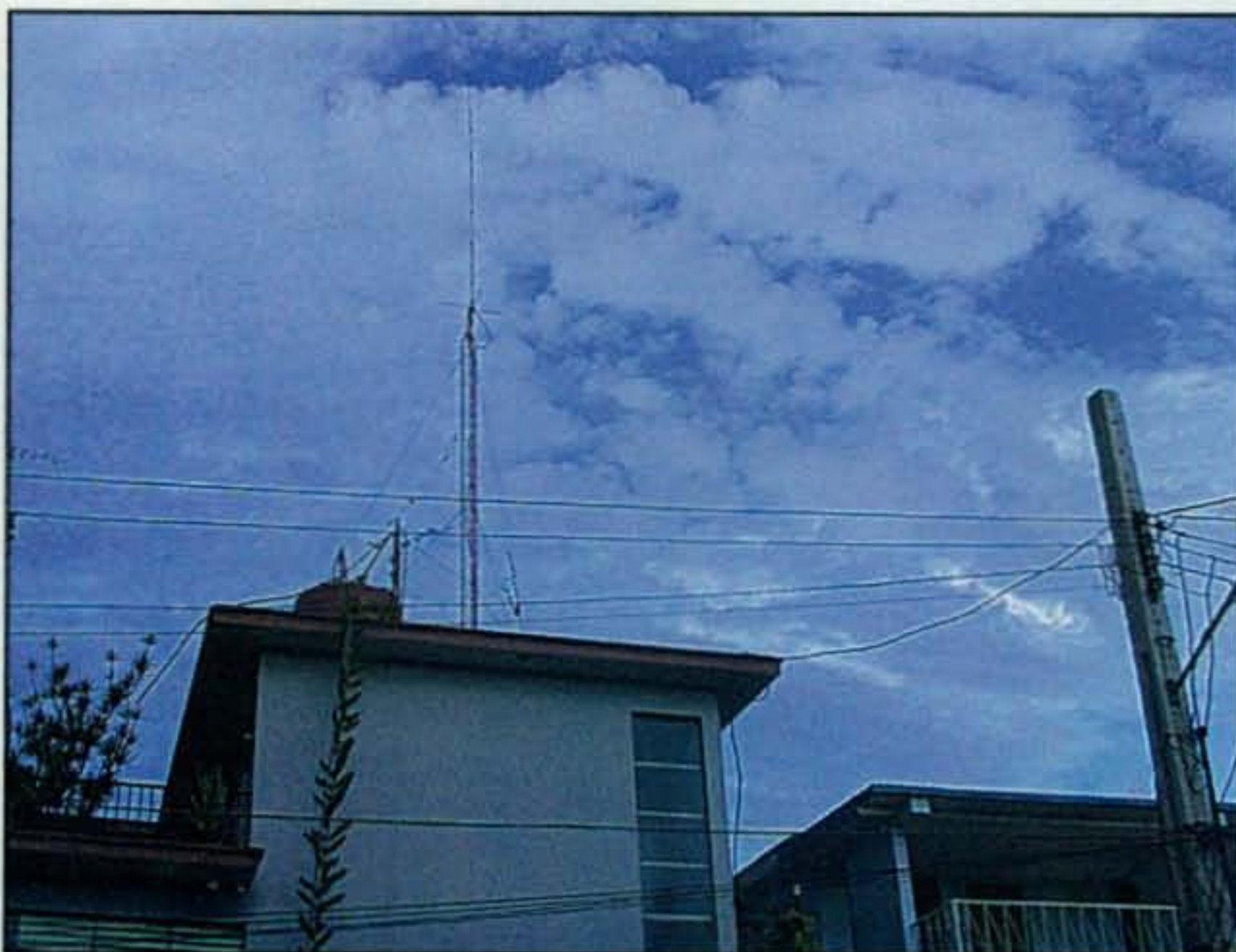
Photo A— Full-size, 2 meter, omnidirectional, vertically polarized antenna at CO2KK's QTH using three 5/8 -wavelength elements. With its estimated 6 dB gain over a dipole, it's my standard of comparison for 2 meter FM work.
